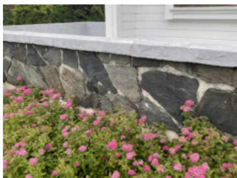
Riss/sprekker.
