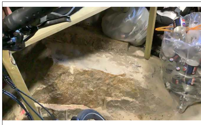
Bod bak carport.
