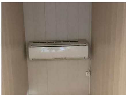
Varmepumpe innerdel.
